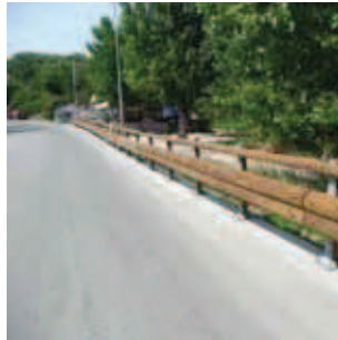
Handrail with half round log diameter 12 cm in 4.00 length - Steel post HEA 100 on steel base
